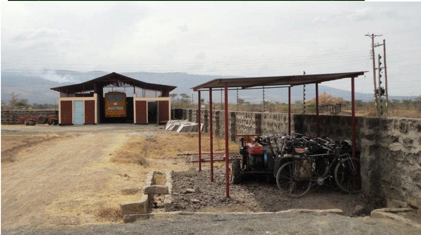
Garage with store and workshop on either side and a shelter for bicycles and the mower.
