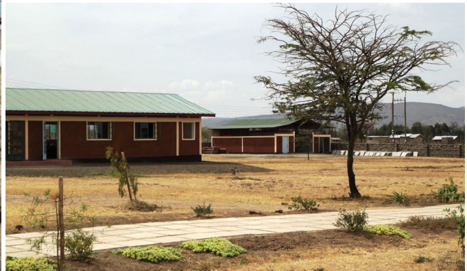
The new classroom block with garage in the background.
