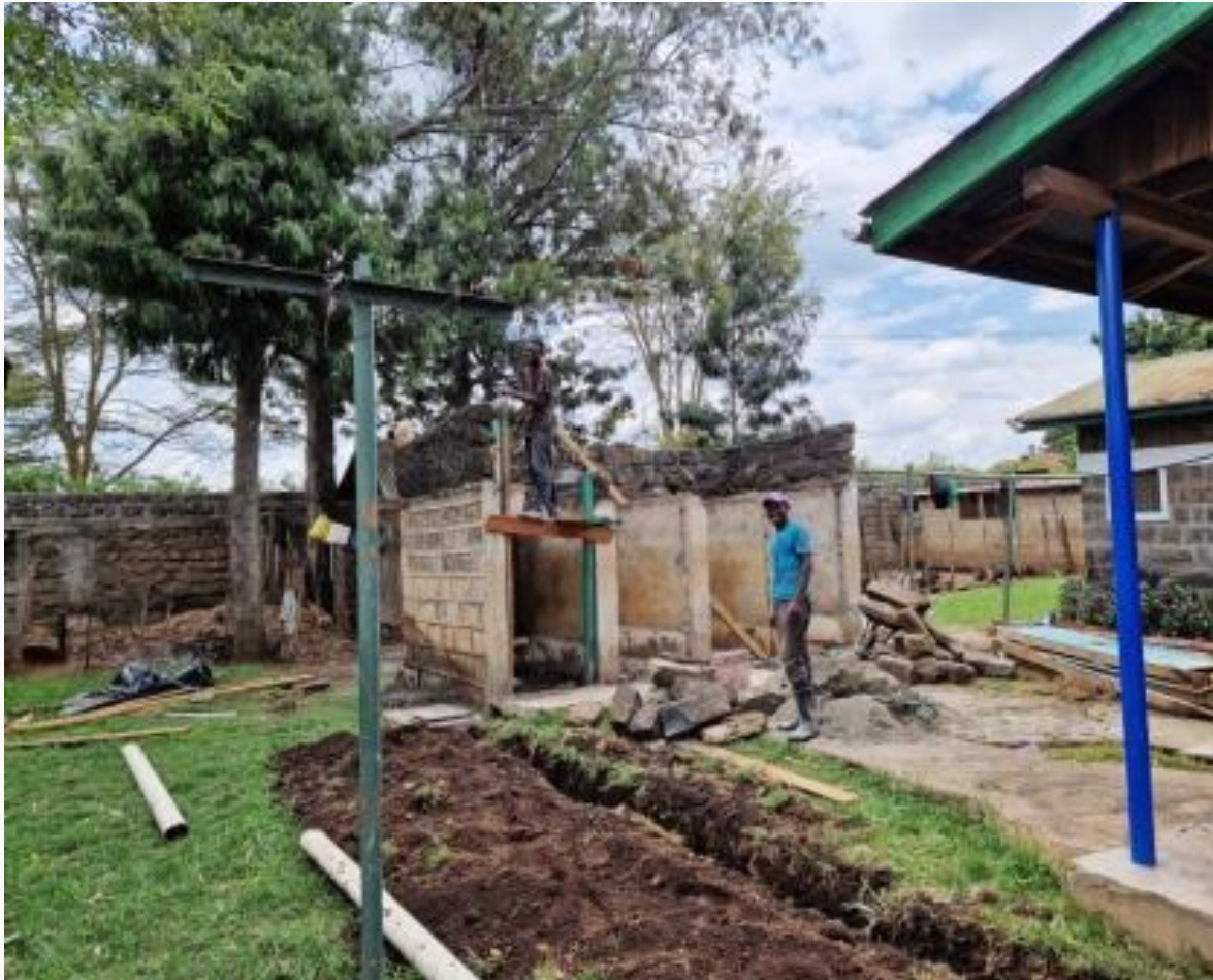
Siting the biodigester, luckily before the rain set in! The level of the loos had to be raised to ensure good flow.
