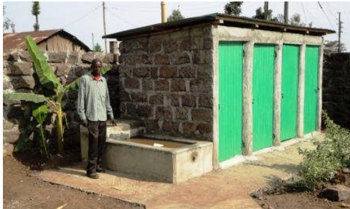
Fred the contractor at the latrine block and basin.
